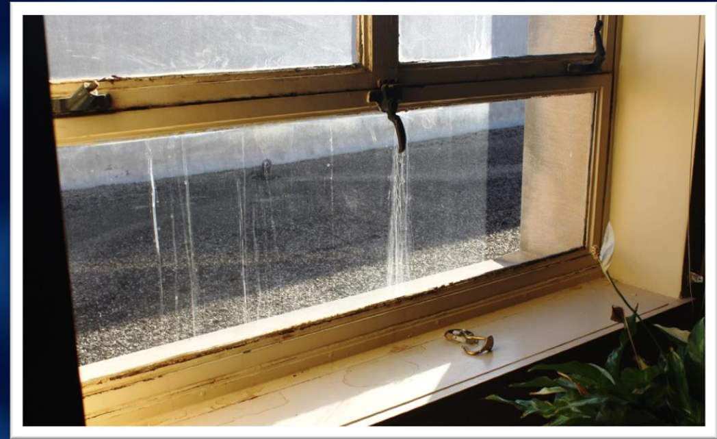
Original, single-paned windows are inoperable, rusted, and leak water and air.
