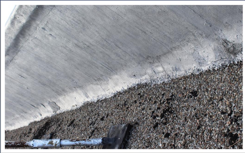
The roof's parapet contains numerous cracks, which allow water into the structure.
